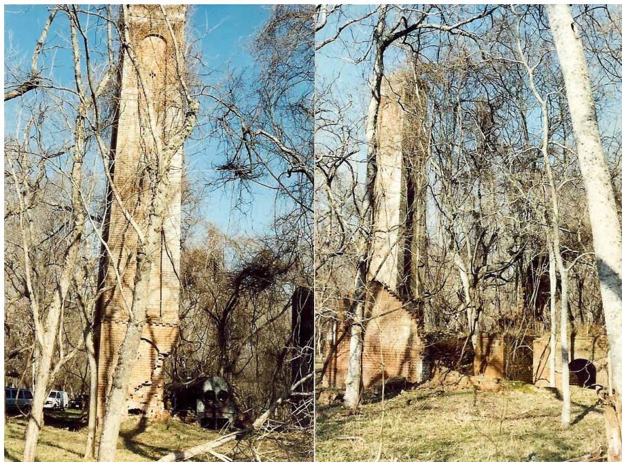
Photos January 1996 Osceola Boiler Chimney ~45' Height (Courtesy W. Sue Gross)
