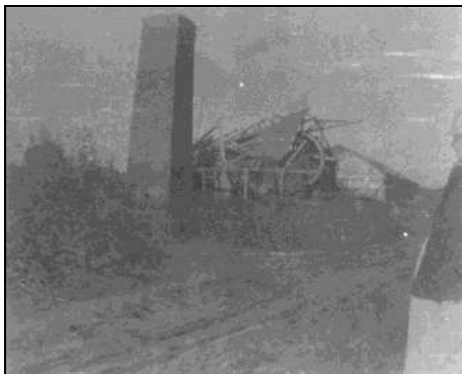
Photo Durazno Sugar Mill Unknown Date Possibly after Hurricane Damage Courtesy of the Brazoria County Historical Museum 29
